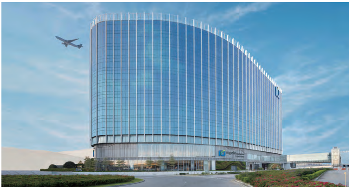
Town gas hot water boilers provide stable hot water supply for the brand-new Regala Skycity Hotel.
