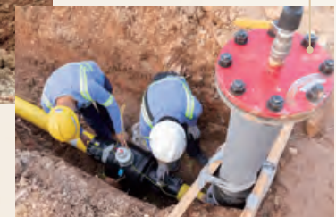
Towngas engineering team worked on the Lok Ma Chau Makeshift Hospital construction site for laying gas pipeline.
